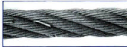
Corrosion, broken wires
