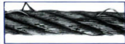
External and internal broken wires. (Valley breaks)
